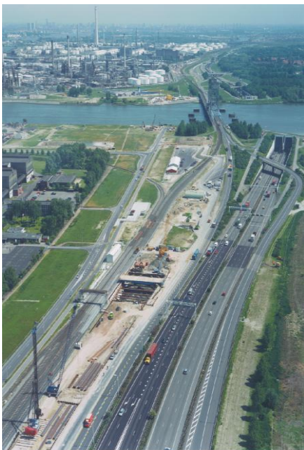
Figure 12 Botlek rail tunnel, under construction
